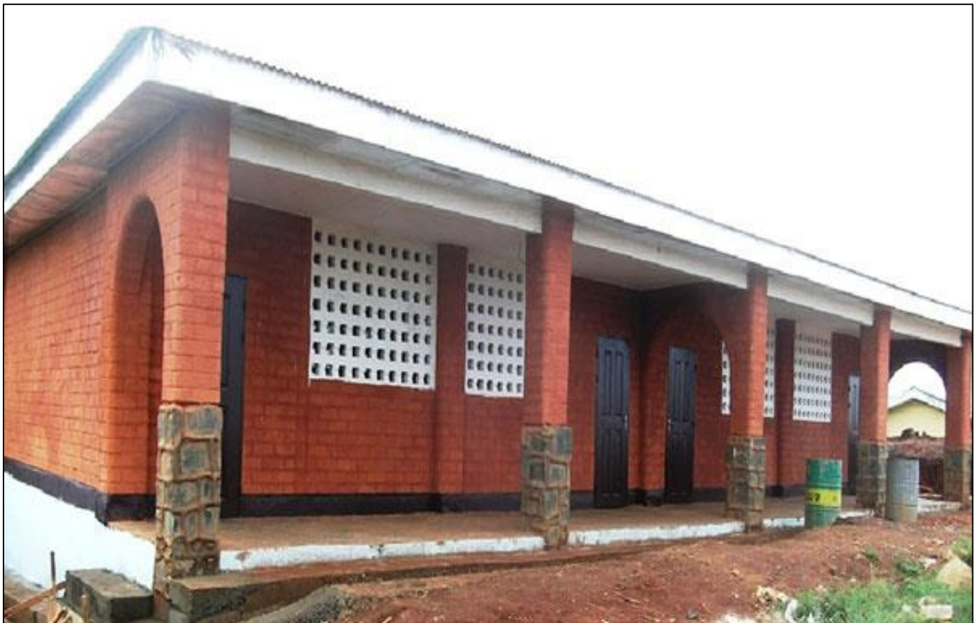
Fig 3 Classroom Construction Project
