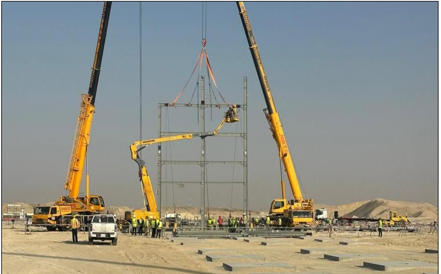
Fig 8 Pre-Assembled structure during installation
