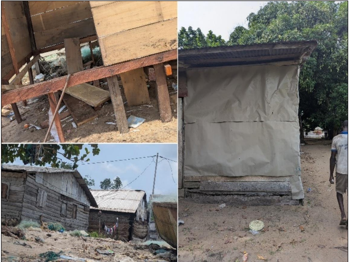
Fig 10 Self-Construction using Recycled Materials
