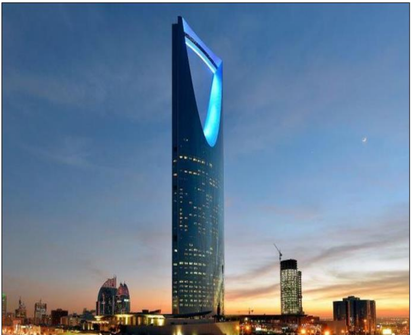
Fig 5The Kingdom Centre in Riyadh, Saudi Arabia, showing a large through-building opening at the top, combined with a tapered form (Ubani, 2020)
