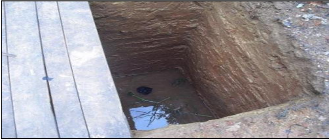
Photo 3 Non-Masonry Septic Tank Photos Kengmoé T Emmanuel, 2024
